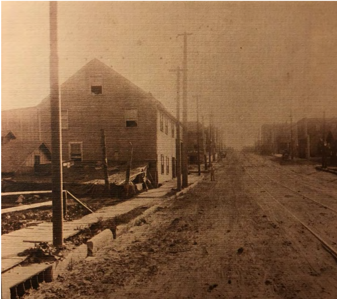
Figure 70. Westport's buildings are mainly two stories in height and roads are unpaved in this photo of Westport Road from the late 1890s. Source: Westport Bank Brochure Celebrating 40 Years of Progress in Westport, Vertical File Westport #2, Missouri Valley Collection, Kansas City Public Library, Kansas City, Missouri.
